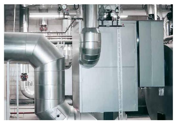
Downstream Vitotrans 300 heat exchanger fitted to a Vitomax boiler
